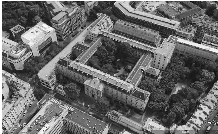
Fig. 6 Aerial view of the École Normale Supérieure building in Rue d'Ulm, Paris (1847, design by Alphonse de Gisors). Image: © Google Earth Pro, © Landsat/Copernicus [accessed 24.11.2022].
