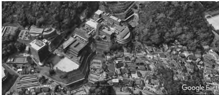
Fig. 42 Example of Cut/fill type: Hiroshima University of Economics (広島経済大学) campus.
