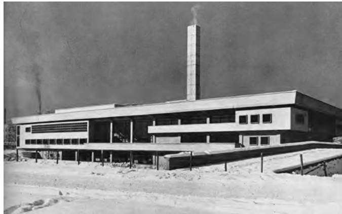
Fig. 69 Hokkaido University, Clark Memorial Students' Hall (design by Ōta Minoru, 1956-59). Source: Kenchiku Bunka (1960-160).
