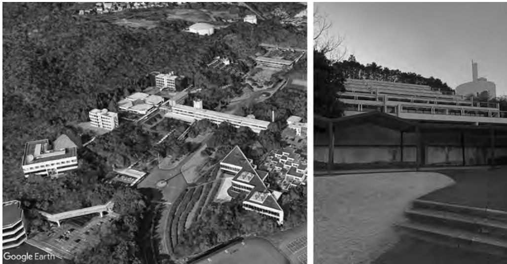
Fig. 58 Nagoya University of Commerce (名古屋商科大学) Nisshin campus (design by Takenaka Corp., 1975). Aerial photo: © Google Earth Pro, © Landsat/Copernicus [accessed 14.3.2023]; right photo by the author, 23.3.2020.
