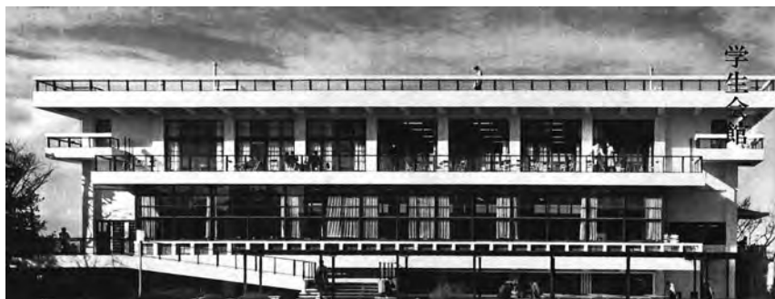
Fig. 67 Meiji University Izumi campus' gakusei kaikan (design by Horiguchi Sutemi, 1960). Source: Kurita
