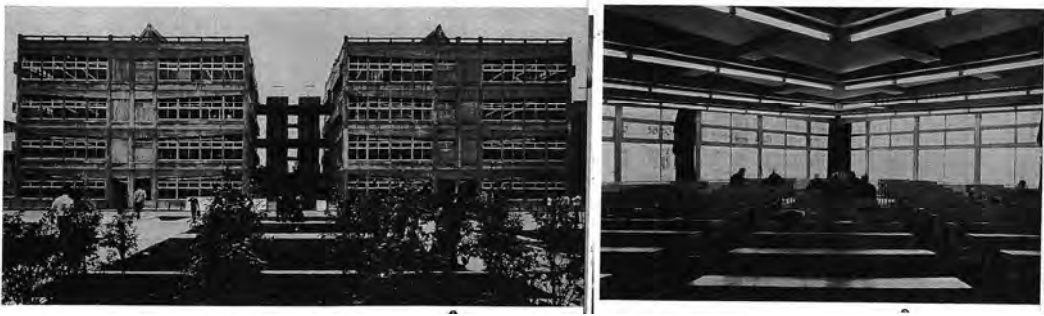
Fig. 53 LRB no. 19 and 20: Waseda University (早稲田大学) Nishiwaseda campus, lecture room buildings (design by Andō Katsuo, 1964). Source: Kenchiku Bunka (1964-208)
