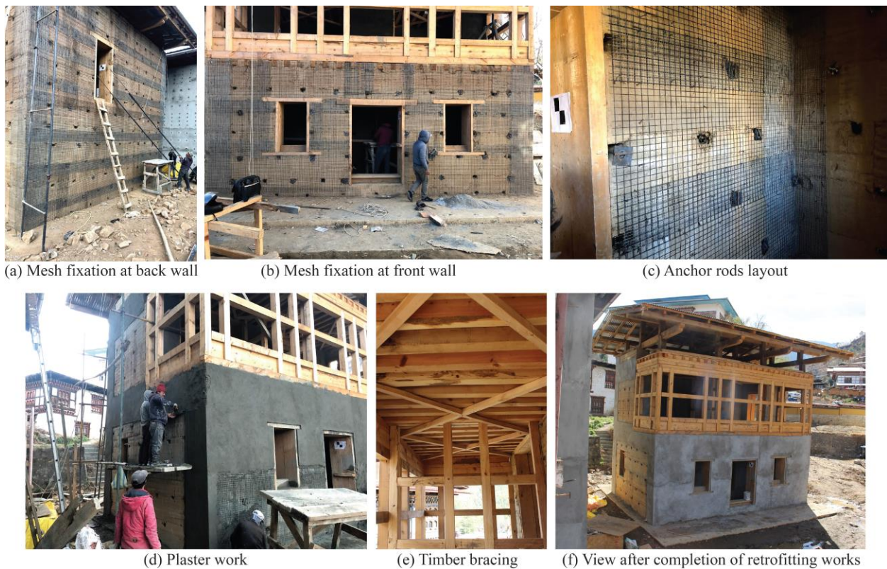
Figure 5.17 Retrofitting details of R-RE-LONG.
