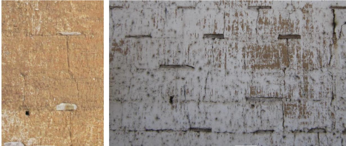
Figure 4.10 Reinforcing method practised in vernacular buildings in Bhutan.
