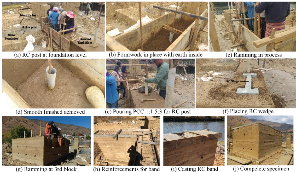
Figure 4.17 Construction process details of New-RE-B.
