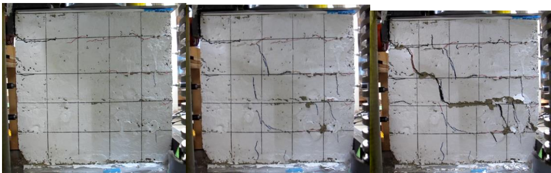
(a) At 5 kN (b) At 5.89 kN (c) At final failure
