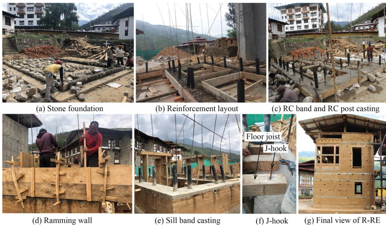
Figure 5.21 Construction process of New-RE-SHORT.
