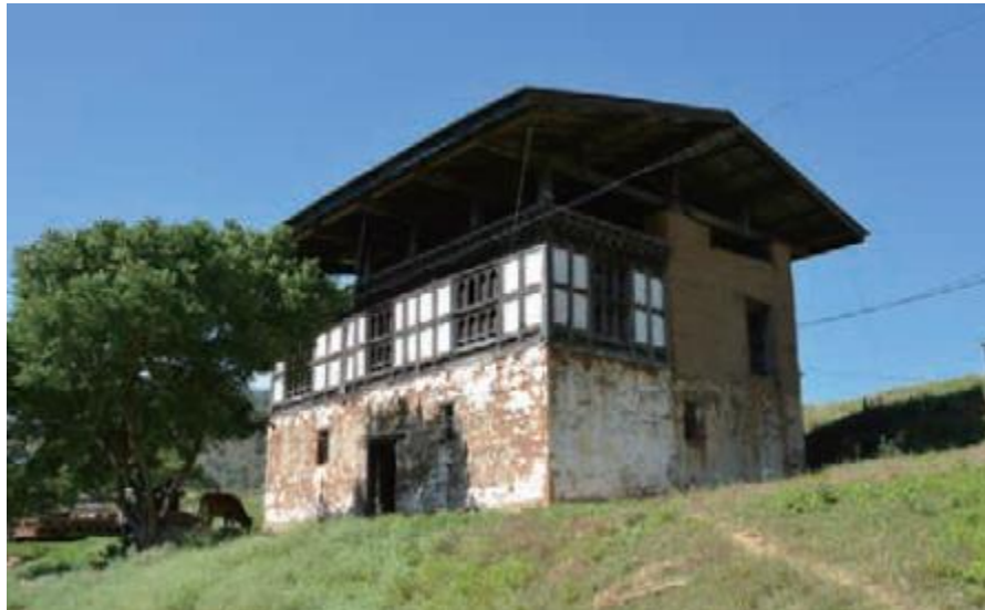
Figure 5.2 Rammed earth house with type D plan (Photo credit: NRICPT and DOC).
